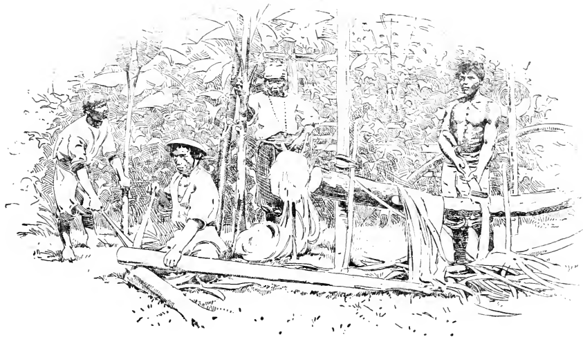
Manila Plant with Cooleys preparing it
